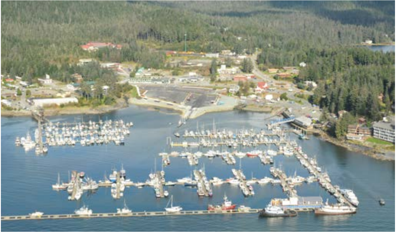
Above: Statter Harbor Launch Ramp Project 2017. Photo by PND Engineers.
