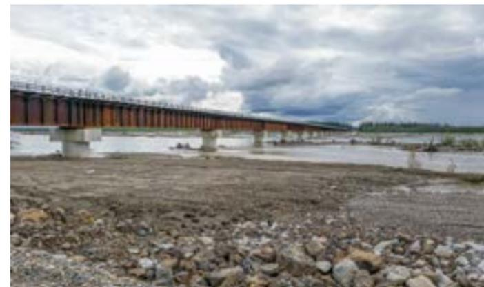
lows near 70 below zero. During construction, piles for the bridge were driven and concrete was placed at 20 below zero in the winter. Ice flows and damming during ice breakup in the spring required the construction causeway and temporary bridging to be removed and replaced.
